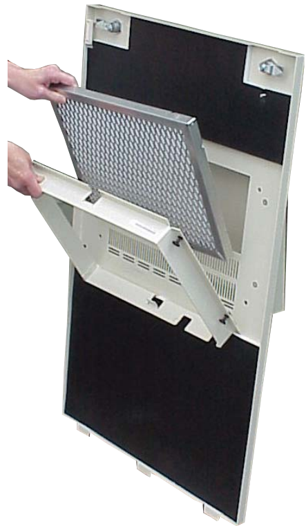
Fig. 7-2, Air Filter Removal, CE-3x2 5K-T
