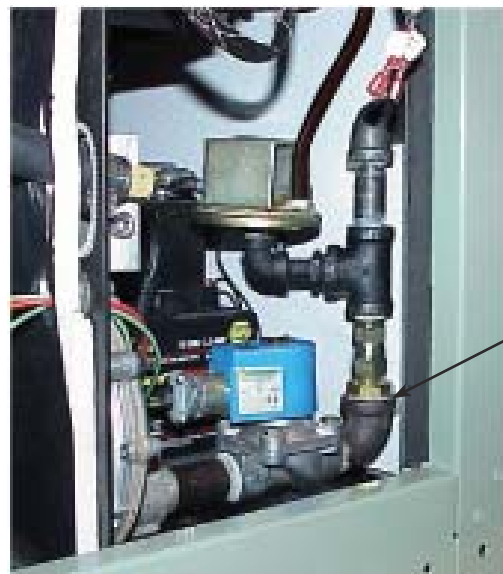
Fig. 7-9, PN-6x-T Switch Assembly Installed
