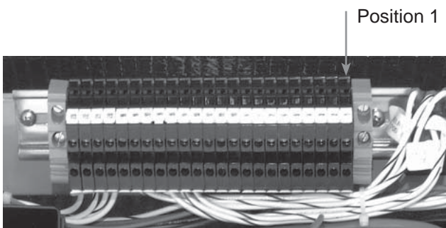
Fig. 3-21, Terminal Block 2 (TB2) Position 1, 5kW
