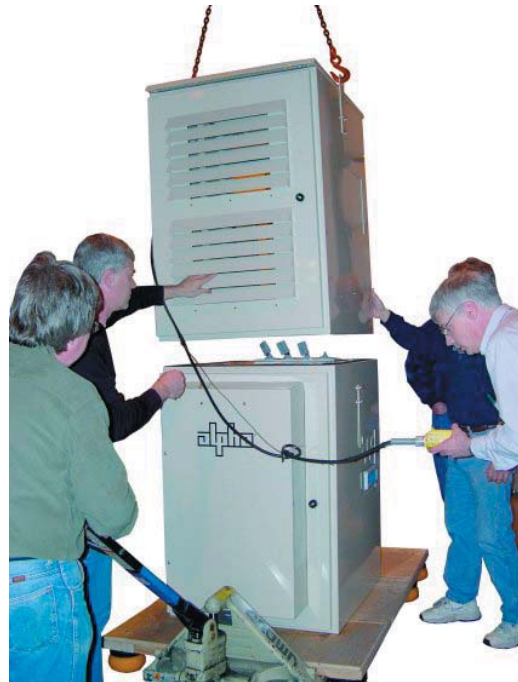
Fig.3-2, Lifting Utility 2 onto Utility 1 (photo is for illustration only)
