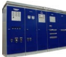
24VDC Rectifiers 24VDC Stabilizers "SASP" OFFSHORE ENG." Clara Complex—Adriatic Sea
