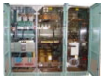
250kVA 115VAC 3Ph. UPS "LITTON" Cruise Ships—USA
