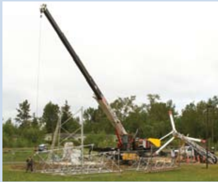
Alpha integrated Solar and Wind Hybrid Power System
