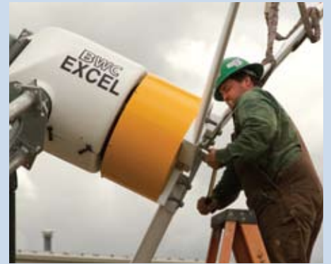
7.5kW wind turbine generates energy in winds as little as 8mph
