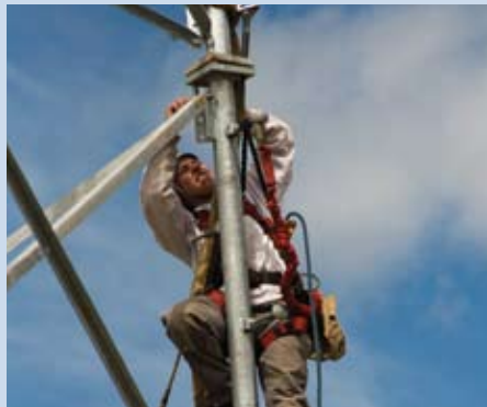
On-site project management
