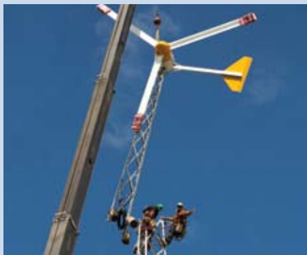
Construction complete in less than 2 weeks
