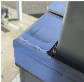
Fig. 9, Reinforcing welds added to Security Bar
