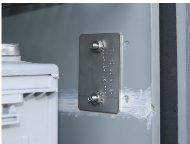
Fig. 5, Reinforcing welds added to Locking Mechanism
