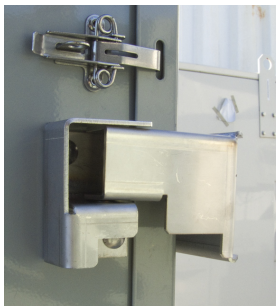
Fig. 5, Reinforcing welds added to Locking Mechanism
