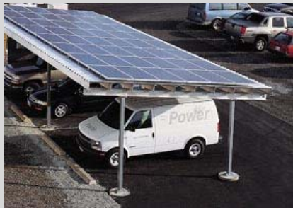
PV Parking structures
