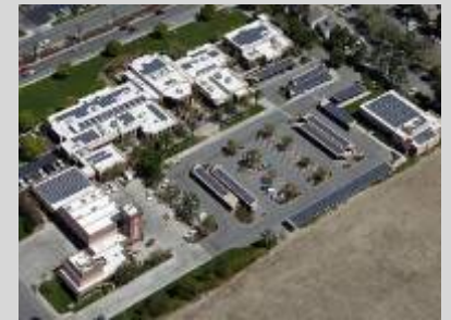
On-Grid Commercial PV
