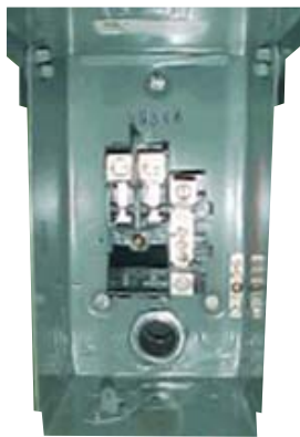
Figure 4-6; BBX 70A (BBX-F12) Square-D, 2-position For single power supply applications
