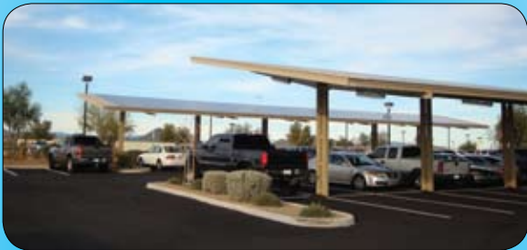
Additional space for modules
