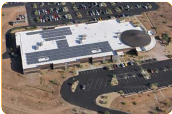
191kW grid-tied solar power system in Phoenix, AZ
