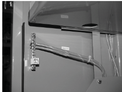
Fig. 3-5, Enclosure Ground Bar
