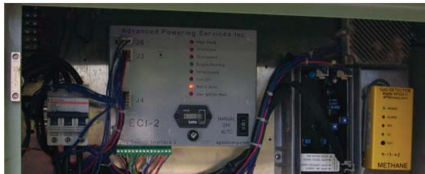
Fig. 2-6, ECI-2 Engine Controller
