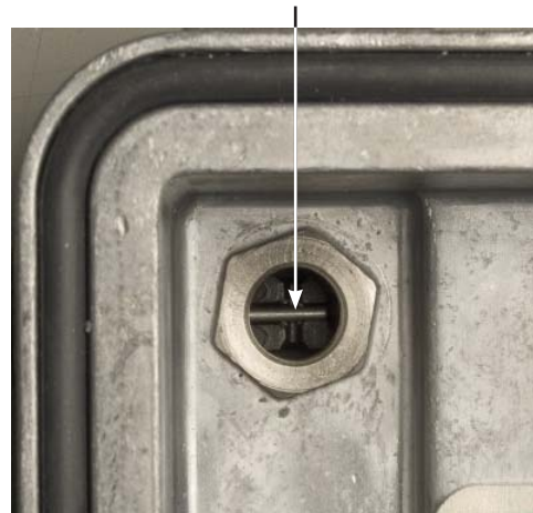
Fig. 2-7, Visible Center Conductor of Installed Connector
