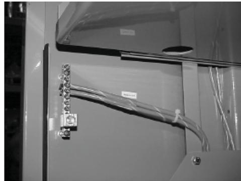
Fig. 3-5, Enclosure Ground Bar
