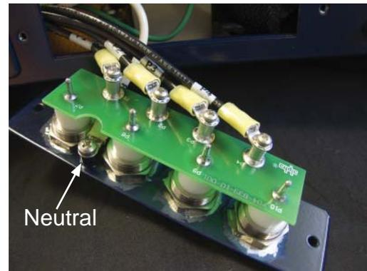
4. Secure the coax cable connector plate to the power supply using the two small bolts. Reconnect line power and switch the battery breaker ON.
