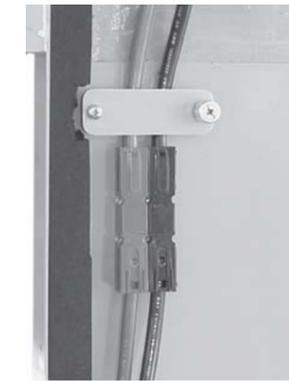
Fig. 9, Cable Retainer
