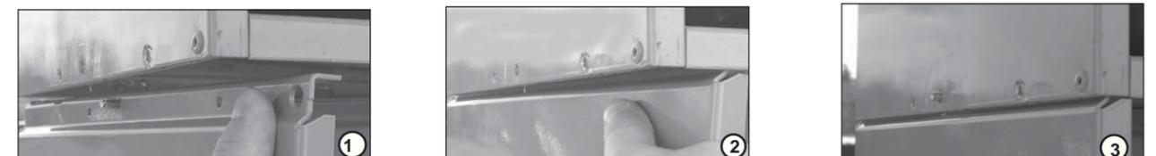
Fig. 3, Maneuver Side of UBE into Existing Enclosure
