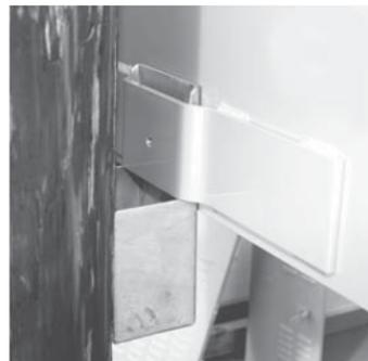
Fig. 6 Mounting the Lower Bracket for Wood Poles
